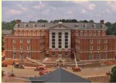
The new Brock School of Business building nears completion.
