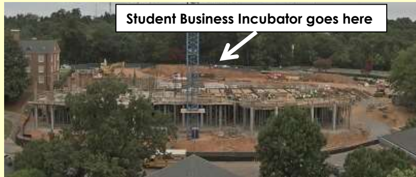
The new Brock School of Business building takes shape.
